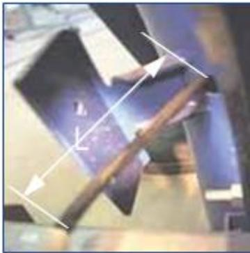
1. Pull the two-core feeder cable with a cable puller through the rail section tube.
